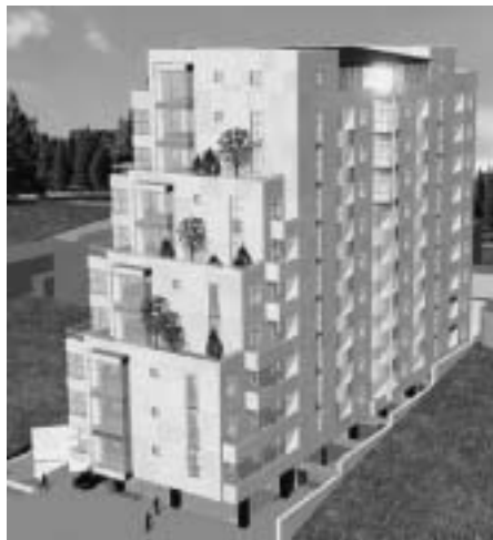
Fig. 3. The view of the 11-story multifunctional residential complex "Cascade" on Demirchian Street in Yerevan
