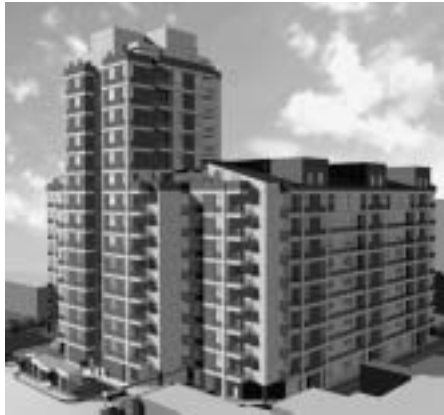
Fig. 2. The view of the 10- and 16-story buildings in the multifunctional residential complex "Our Yard" on Rostomi Street in Yerevan
