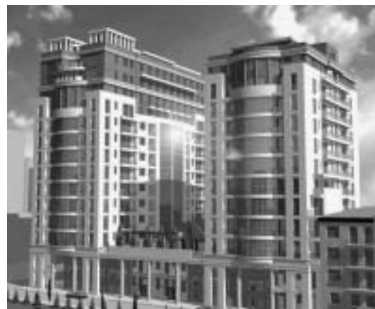
Fig. 5. The view of the 13-story and 11-story multifunctional residential complex on Arami Street in Yerevan
